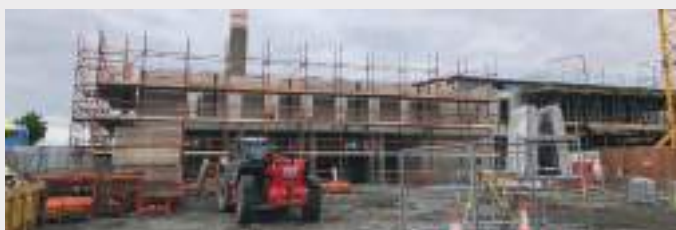
Lidl Ballymun, NordMende Walls Construction
